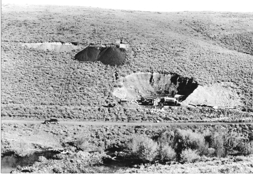
Figure 81. Bloomington Canyon, view north, showing Bloomington Creek, compressor equipment in an old road-metal quarry, and the dump at No. 14 South incline, 1944. Photo from Wyodak, 1944.
